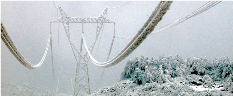
Icing on power network cables ↪ galloping (wind-induced instability)
